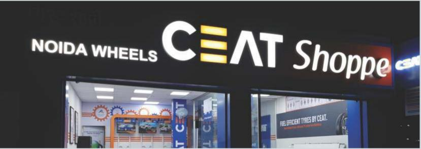
Entire Facade was cladded with ACP. Dealer name was router cut in ACP and lit from inside. Brand name was made in acrylic letters with leds inside and sides were blocked using blockout film. 3M Coloured vinyl was used to achieve brand colour.
